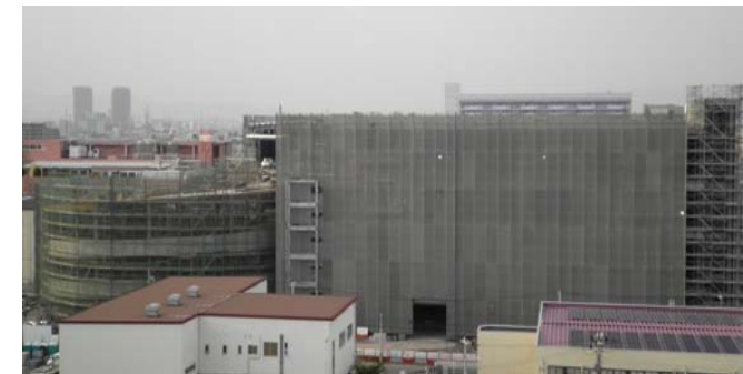
New Distribution Center under construction (from the rooftop of the current Amagasaki DC)
